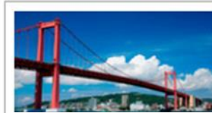
Wakato Bridge connects Wakamatsu and Tobata
